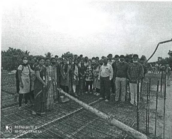
RCC laying using booms, Siddhartha Medical College, Tumkur
